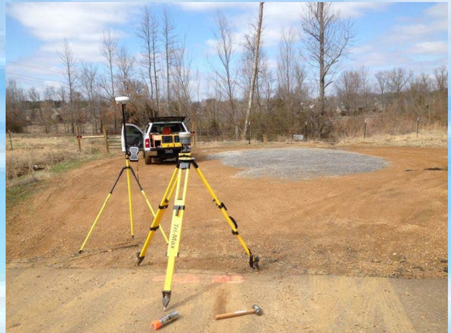
GPS RTK Base Station Setup
